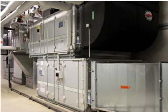
Image caption: In the past, HVAC installations used to be sized overly generously; today, their power output is on the lean side. However, on-demand control and free night cooling make it possible to save energy. Source: Siemens AG
