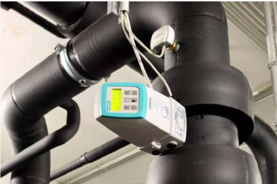
Image caption: Upgrades with cooling and electricity meters is required in order to continuously record a chiller’s energy efficiency.
