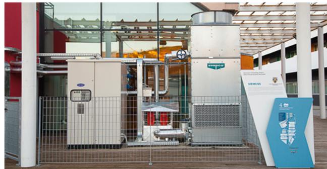
Absorption chiller that converts turbine waste heat into cooling energy
