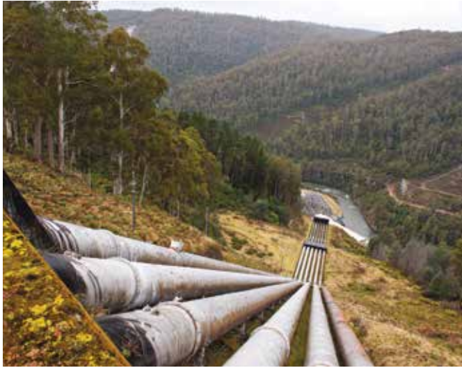
Tarraleah power station
