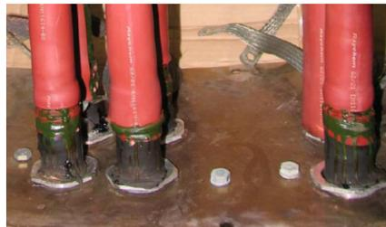
Figure 2: Thermal damage to cables
