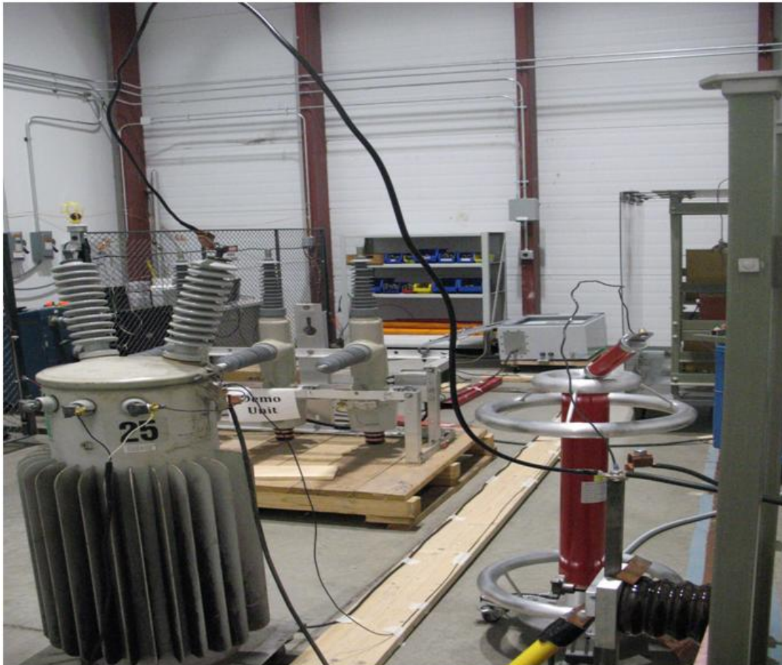
Test Setup with the transformer
