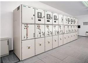
NXPlusC medium-voltage switchgear with Siprotec 5 protective relaying
