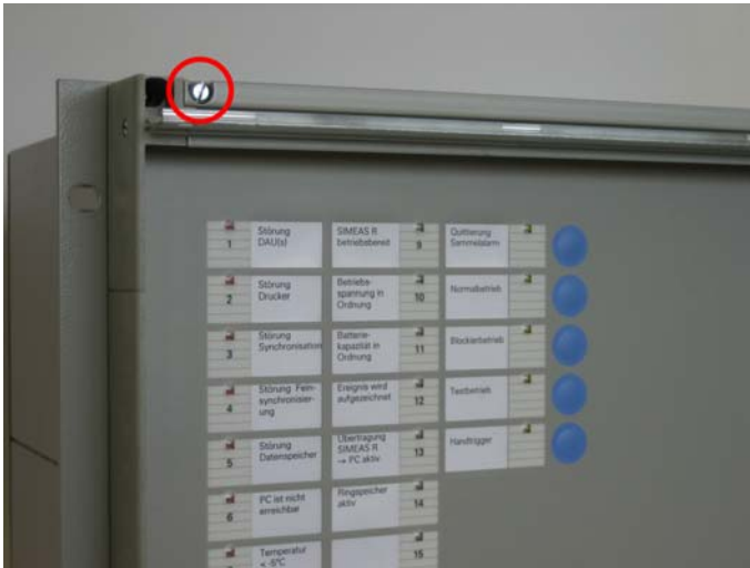
Figure 38: Remove the cover
