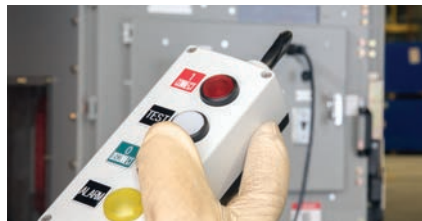
SIERS for medium-voltage motor controllers
