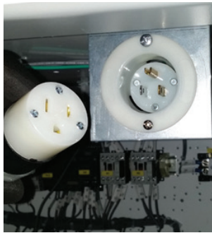
Figure 2: Flanged inlet type 5-15P (on right) for connection to external 120 Vac power source extension cord receptacle type 5-15R (on left) (optional)
