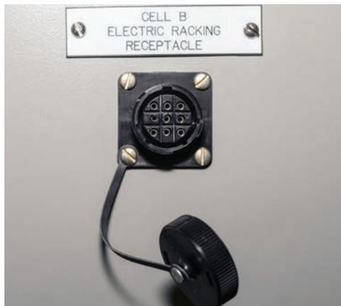
Figure 6: Connector for control pendant cable connection
