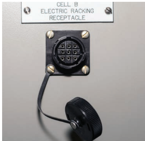
Figure 6: Connector for control pendant cable connection
