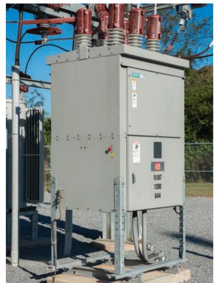
A recloser is distinguished by having a mandatory automatic control and protective device, but this is not significant as most high-voltage circuit breakers used in utility distribution systems have protective relays with similar (or even identical) functionality.
