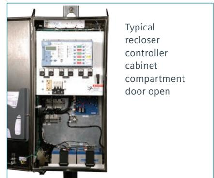
Typical recloser controller cabinet compartment door open
