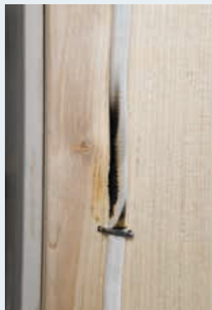
Damaged wiring
