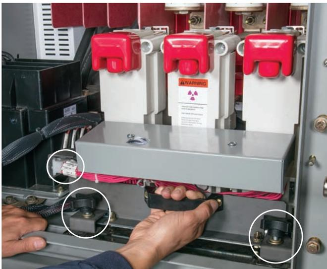
In either the drawout configuration of the Series 81000 or the fixed-mount installation of SIMOVAC, the required functionality and interlocks required by the UL 347 standard are maintained.
