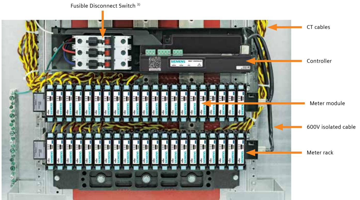
Figure 2 SEM3™ - Embedded Micro Metering Module™ components in a panelboard
