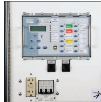
Type 7SR224 control and protection relay (three-phase)
