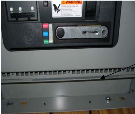
Figure 7: Front view of Mounting Base
