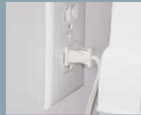
Pushing furniture against cords plugged into outlets
