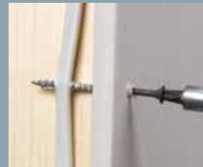
Accidentally piercing electrical cable behind drywalls with drill bit, nail, or screw
