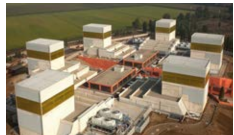
The Eni Green Data Center in Ferrera Erbognone
