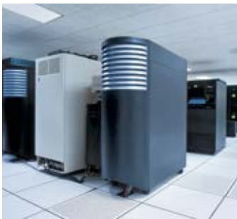
A bundled, consistent power supply portfolio from high to medium and low voltage
