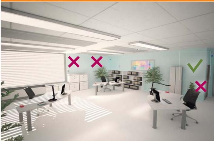
To ensure optimum acquisition of the room temperature and thus energy-efficient operation and enhanced room comfort, the following rules should be followed when mounting GAMMA room temperature controllers:
