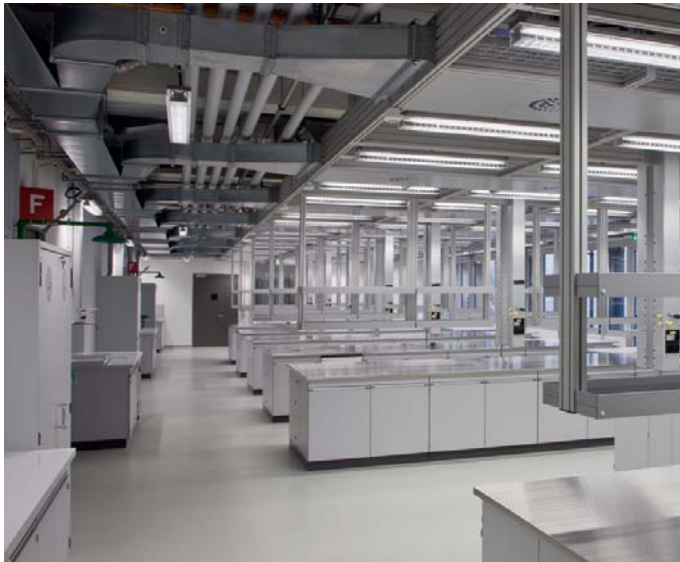
A laboratory with variable volume flows at Dow Europe in Horgen
