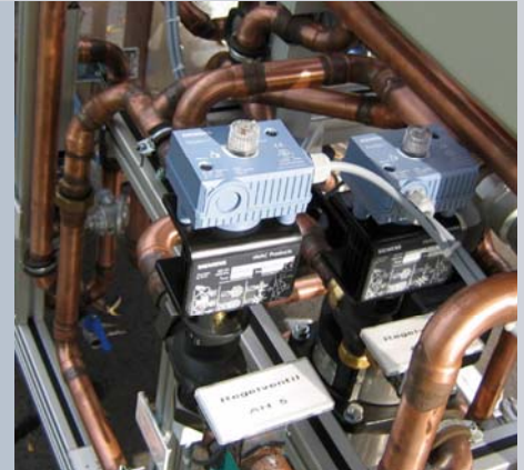
Two magnetic control valves type MXG461 connected in parallel ensure fast and accurate control of preset parameters
