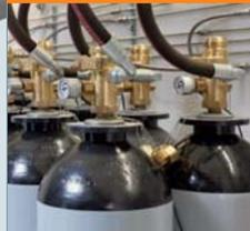
Recommended for medium- to large-sized data centers, Sinorix CDT technology discharges gas into the flooding zone at constant mass flow during the entire flooding time – eliminating the peak at the beginning of the discharge. This lowers the maximum noise level and the size of the overpressure flaps can be reduced by up to 70%.
