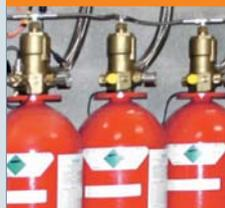
For small- to medium-sized data centers, Siemens recommends Sinorix 1230 based on 3M™ Novec™ 1230 Fire Protection Fluid. It floods the room within 10 seconds and starts extinguishing before any electronic equipment is severely damaged.
