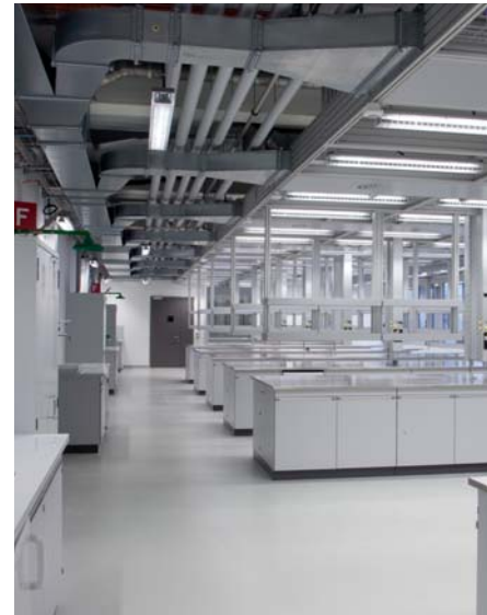
A laboratory with variable volume flows at Dow Europe in Horgen, Switzerland.
