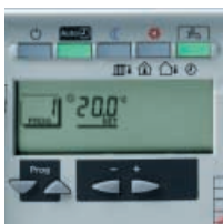
Push-button setting of setpoints, time of day, holidays etc.
