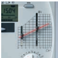
Established analog heating curve setting facility
